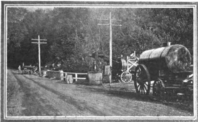
Resurfacing old roadway with a coat of tar oil and stone screenings
